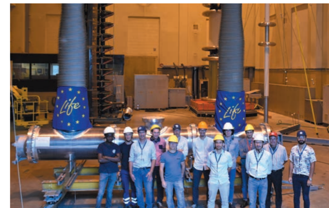
5. LifeGRID team in front of the g 3 GIS circuit breaker that successfully achieved the test phase
